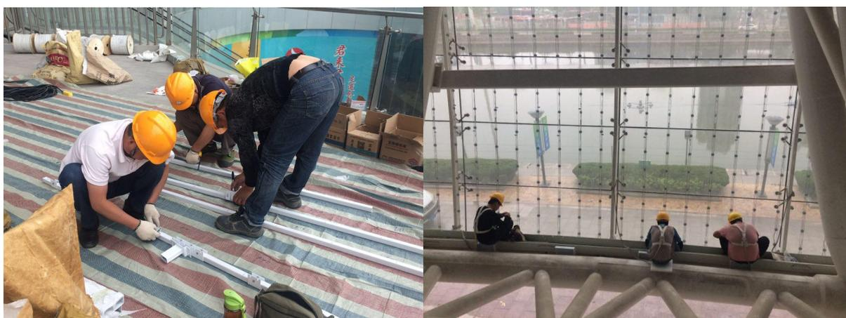
Figure 3: photos shows the worker doing the installation for the LED mesh screen on site.
